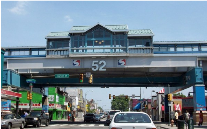
SEPTA Market-Frankford Line The "L" 52nd & Market Street, Philadelphia 2016 D Cramer photo
