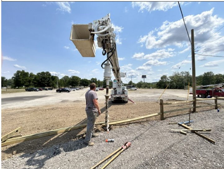
Fence post installation at Ellis Stop 7-16-24 Scott Becker photo
