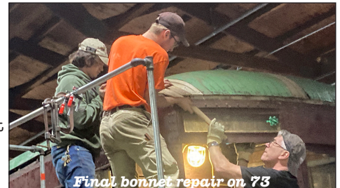
Final bonnet repair on 73
