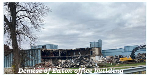
Demise of Eaton office building
