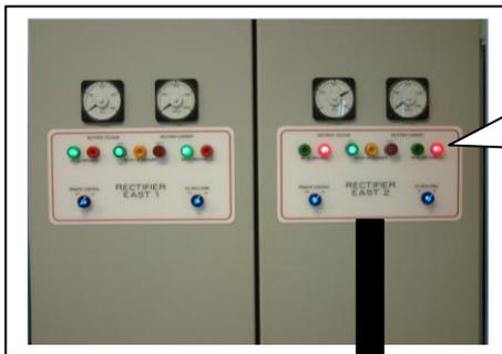
The rectifier that is being used is indicated by the two red lights as shown here. Turn line power on and off on this rectifier.
