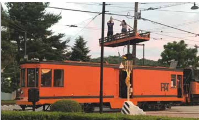
Our bundles of energy work day, evening and night to keep the museum humming along. Here Jeff King runs the line car while Laura Wells and Kevin Zebley change the bulb in the street light.
