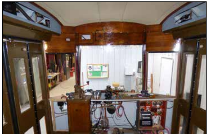
Work progresses on the interior of West Penn 832 as the project gets into its final stage. Photos by Bruce Wells.
