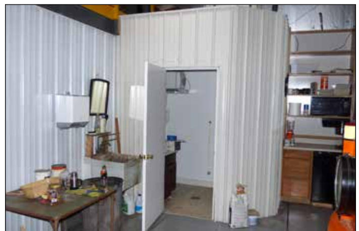
Incremental progress on the shop wash room is seen in context to its location with the mezzanine to the left and West Penn 832 on the right. Photo by Sarah Wells
